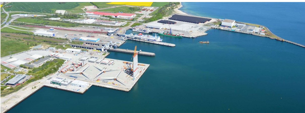
Figure 2.9. Mukran port in Baltic Sea, Rügen, Germany. Source: [29].
