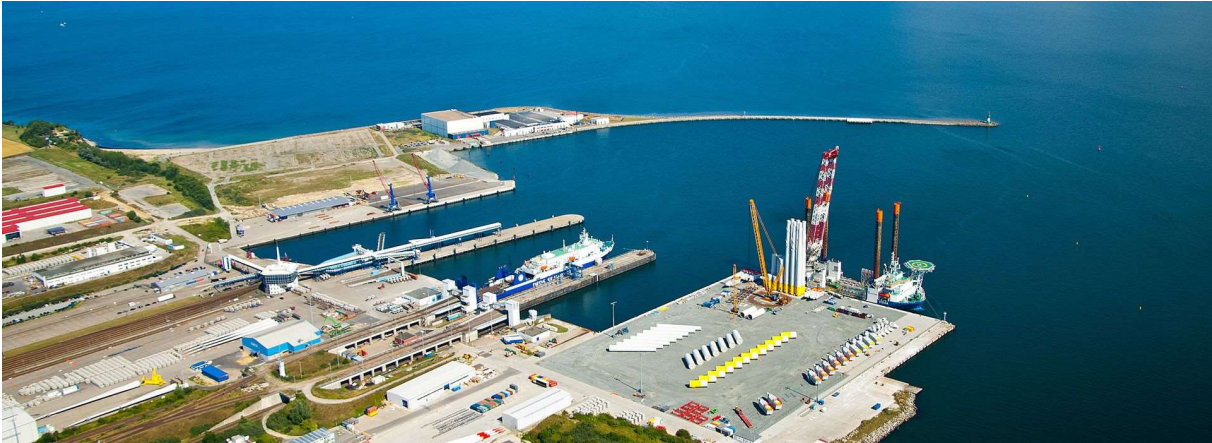
Figure 2.8. Mukran port in Baltic Sea, Rügen, Germany. Source: [29].
